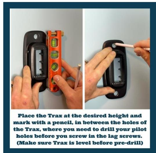
**Place the Trax at the desired height and mark with a pencil, in between the holes of the Trax, where you need to drill your pilot holes before you screw in the lag screws. (Make sure Trax is level before pre-drill)**
