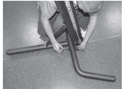
**10.** Attach back tubular floor brace to post with (2) hex head bolts  $3/8'' \times 3/4''$  long and (2) lock nuts. **DO NOT TIGHTEN FULLY AT THIS TIME.**
